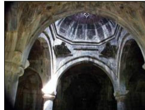
The impressive **Hamazasp gavit** (1257) with an adjacent chapel, is just above the depository gallery. From an engineering standpoint is remarkable, it being the largest gavit in Armenia, and surviving numerous earthquakes with little damage. It is rectangular in plan with four identical abutments and columns supporting sectioned vaulting leading to the central octahedral open dome. The ceiling is divided into nine panels
