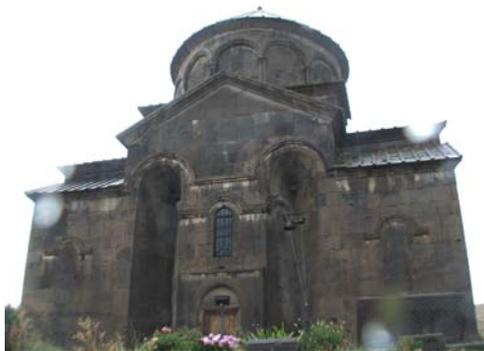
It also features an early use of niche buttressing, which distributed the weight of the dome to the corners of the outside walls, where the building was strongest. The niches are topped by scallop arching, each one in a different design.
